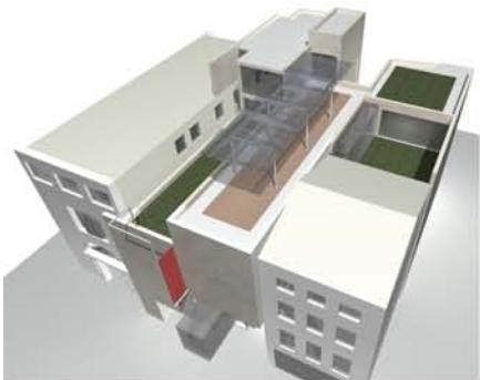
ROOFSCAPE Timber decked viewing terrace with photovoltaic canopy
